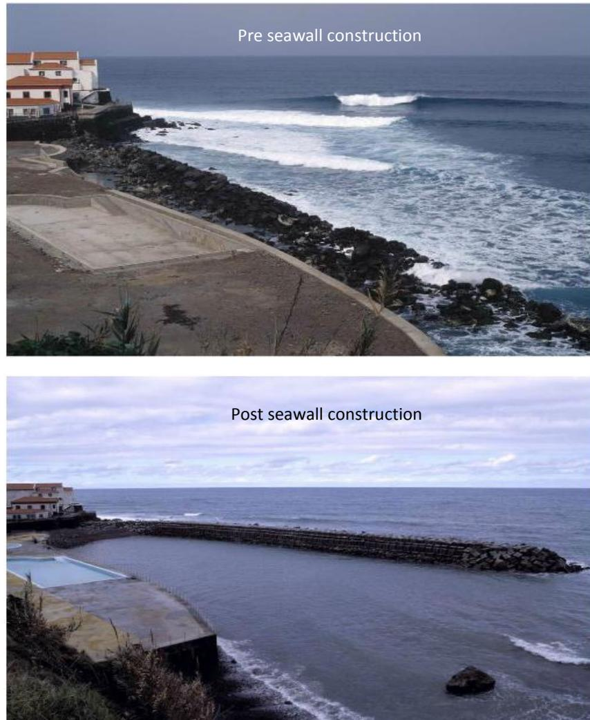
**Figure 4: Photos showing the destruction of the wave at Ponta Delgada on the island of Madeira, Portugal. The top photo shows the wave prior to the construction of the seawall and the bottom photo shows how the wave has been affected post seawall construction. The pool that the seawall was built to protect is can be seen to the left in each photo. Photos from Henry, (2011).**
